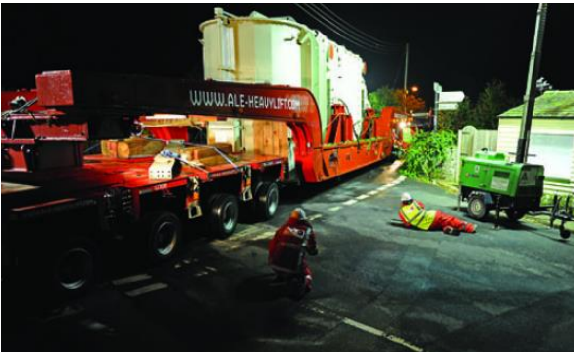
Image from the London Array Limited website showing delivery of an onshore substation transformer across a rail bridge in the village of Graveney, Kent.
