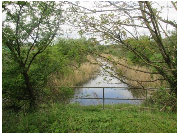
Photograph 21 Alternative view of Bathside Culvert.
